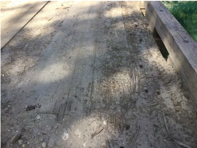
Planks wearing at approaches
