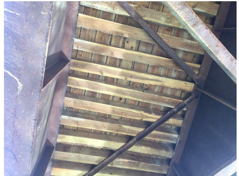
Ties and subdeck condition from underneath
