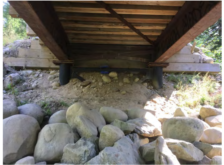
Left Bank Abutment when facing downstream
