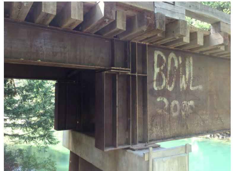
Main span to jump span bearing seat
